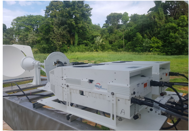
Field installation of IBUC G model
