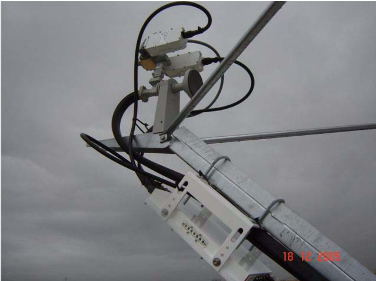
Figure 3.4 Actual Installation of Rx 1+1 System on Antenna Boom Arm
